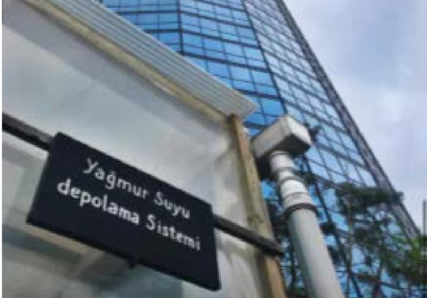
A rainwater storage system
